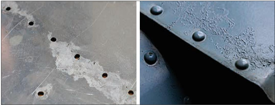
Figure 10. Pitting and filiform corrosion visible along rivet lines and the aluminium skin surface of a military aircraft. Image source: Aero Corner.
